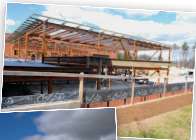
Construction on the New Emergency Department
