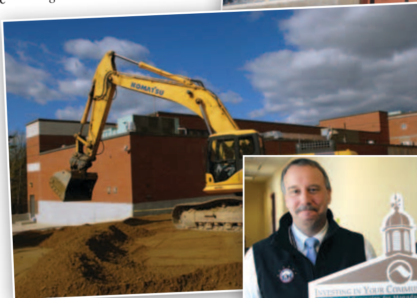
Construction on the state-of-the-art surgical wing
